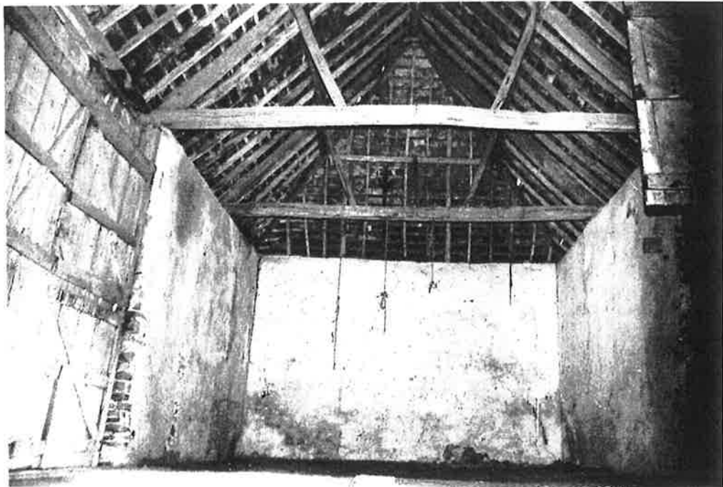
First floor showing the plastered walls
